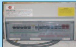
New Style RCD Fuse Box
